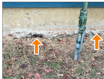
A. Item 2 Perimeter beam, right side (facing front)
