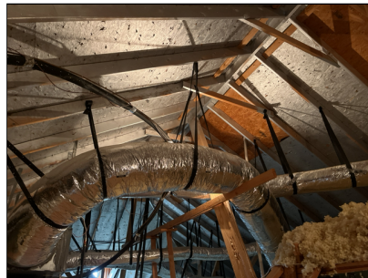
D. Item 2 View of roof structure in attic
