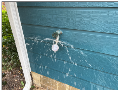
A. Item 1 Hose bib, right side (facing front)
