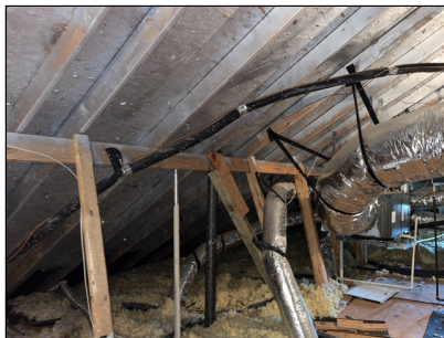
D. Item 3 View of roof structure in attic
