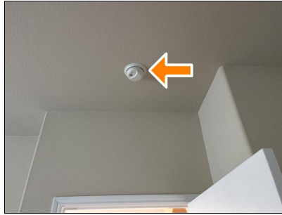
B. Item 1 Smoke detector, master bedroom
