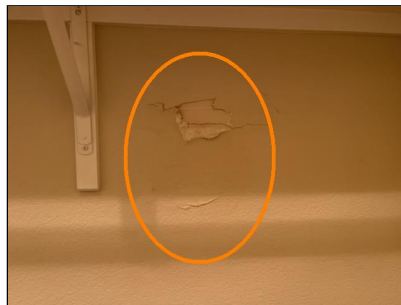
E. Item 10 Wall, utility room
