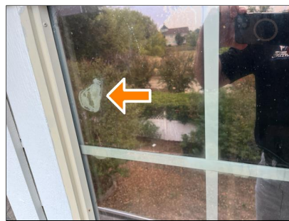
H. Item 1 Window in dormer at rear of home
