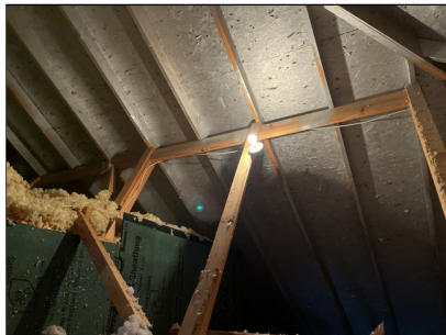
D. Item 1 View of roof structure in attic
